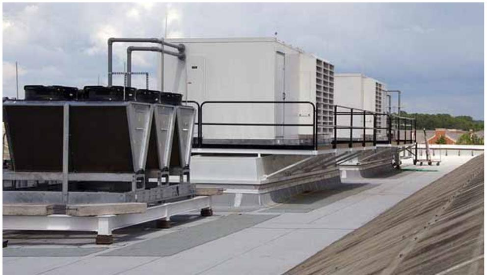
Seresco Technologies has recently introduced the Protocol, which uses up to 85 percent less refrigerant than a traditional dehumidifier. Instead of refrigerants and copper piping, the process uses glycol, heat exchangers, and PVC piping, which significantly reduces the environmental impact and continually rising refrigerant and labor costs associated with dehumidifiers using a full charge of refrigerant. (Photo courtesy of Seresco Technologies, Ottawa, Ontario.)
