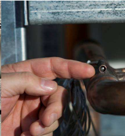
Figure B-5. Sensor in well
