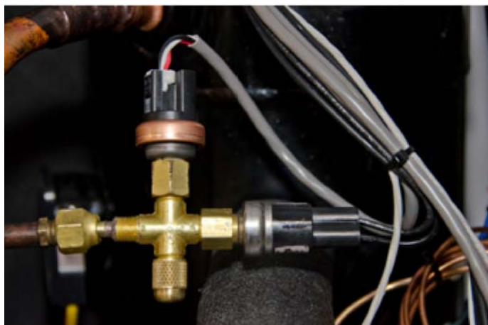
Figure B-7. Pressure switch (2-wire) and transducer (3-wire)
