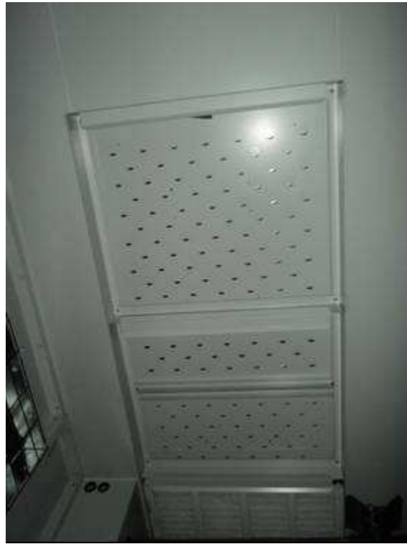
Figure H-3. Outdoor Air Filter Box
