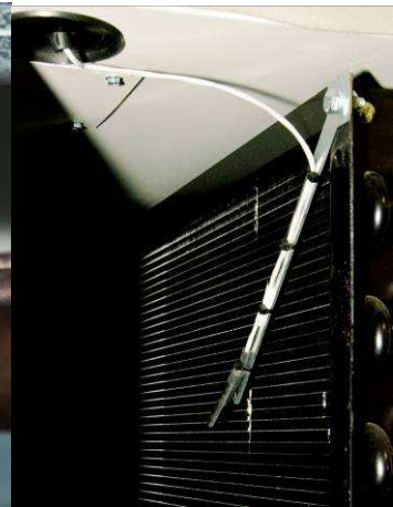
Figure B-6. Evap coil sensor
