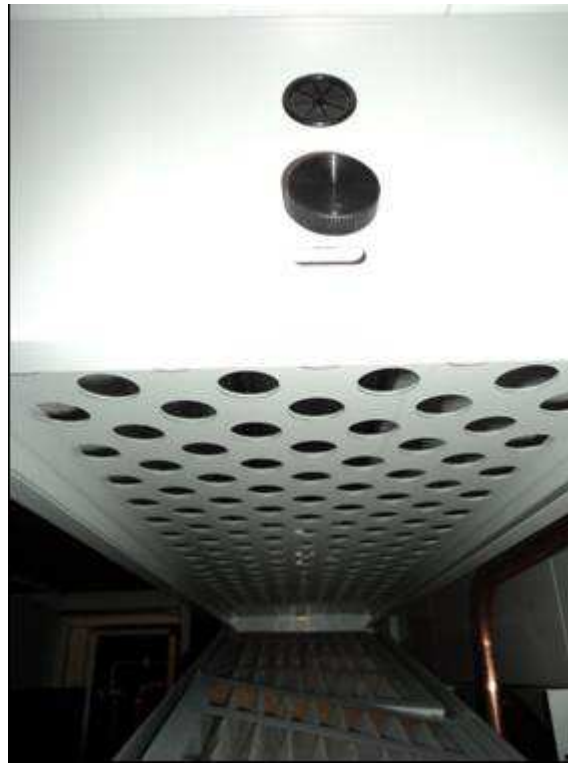
Figure H-2. Outdoor Air Filter Box
