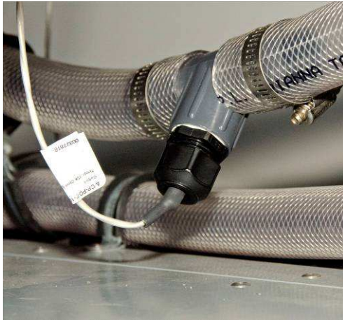
Figure B-4. Pool water sensor
